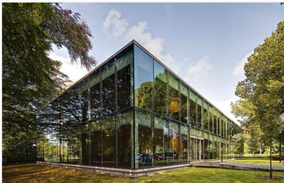
Renovatie BOM Tilburg
